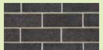
Natural colour mortar with rolled joints
