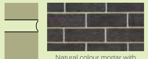
Natural colour mortar with rolled joints
